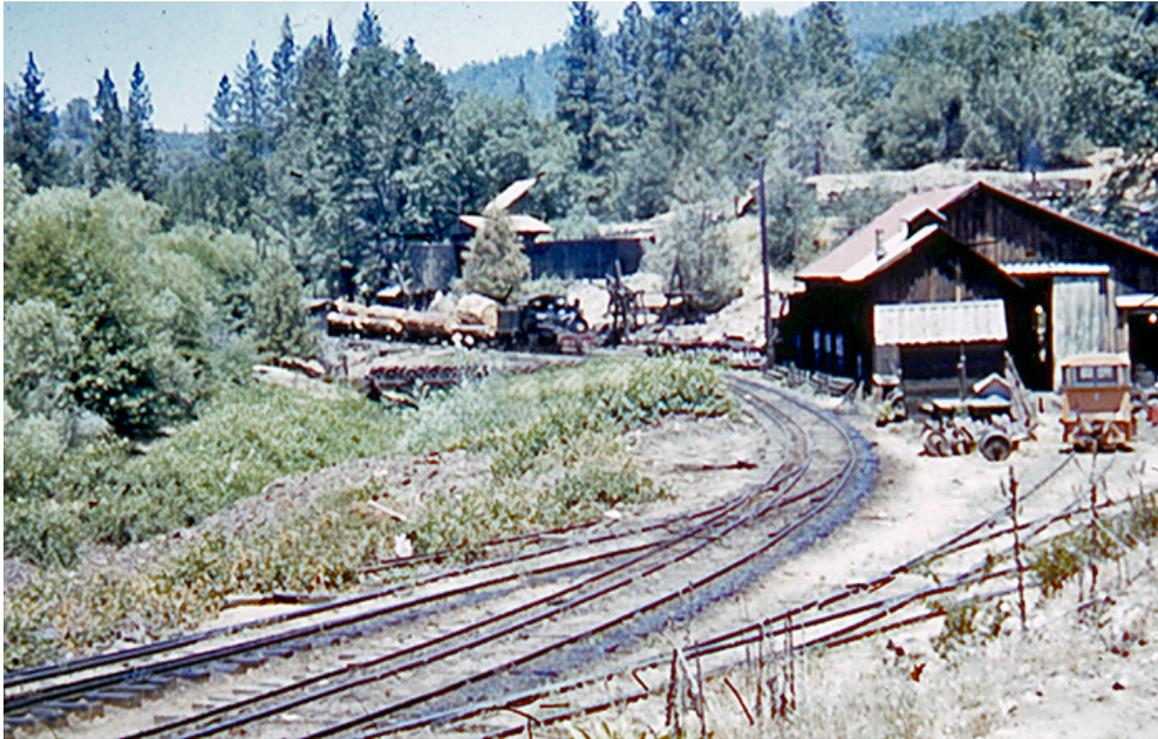
As the train first appeared, many details of the area could be seen. Gas switcher no. 1 is at the right; the platform and high pressure water nozzle for washing empty log cars was at its left. Behind that was the blacksmith's charcoal storage shed.
