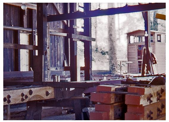
Coming back through the shops, I went up into the shop that once was the original engine house. There, I photographed a new beam being installed on a log car. Other new beams, complete with hardware, were piled and awaiting installation. I did not record what caboose was in the background.
