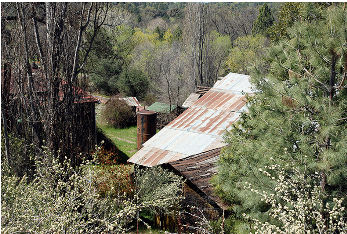
A slightly different view of the area behind the 3 stall car shop. The charcoal storage shed is at left center. The railroad's main line into the yards was on the far side of the shed.
