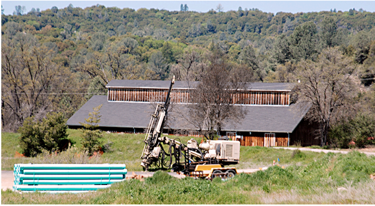
Bell's old WS&CV engine house. The Me-Wuk tribe may be using it for storage.
