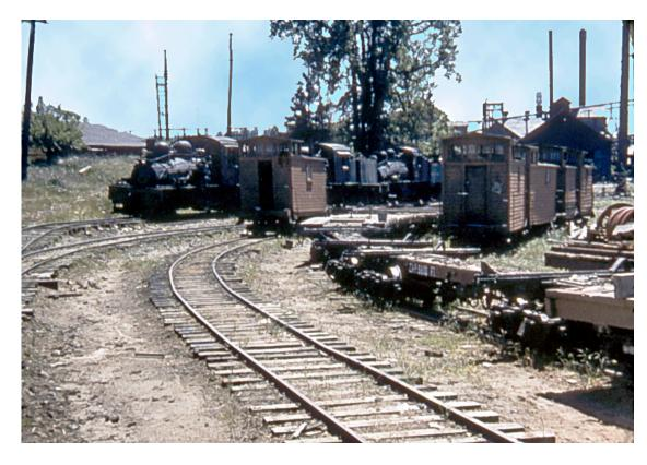
This is the lower yard. All this equipment is 3 foot narrow gauge. Three Shays are on the left (from the front: #8, #9, and #12). Five cabooses are visible but I didn't record the numbers. Through the middle is a mixed string of cars. From the right: a logging flat car (with part of a bunk on it perhaps), two Swayne type
