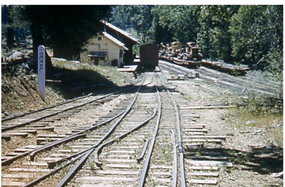
This is looking down from the wye. First track on the left is the third leg of the narrow gauge wye. Second track on left is a siding. White building on left is Dispatcher's Shack. A reefer is beside the woods warehouse for loading. A work train with 4 tractors on 4 equipment flats is on the main line and two flat cars are on the siding next to it.
