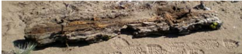
Photo B (above) and Photo C (left): Surviving railroad ties with spikes and spike holes allowed the gauge of the line to be established at 36" between the rails. Photo B: April, 1010, Photo C: June, 2006 by the author.
